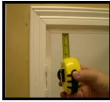
Measure Right & Top frame for spacing.
