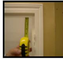
Measure Left & Top frame for spacing.
